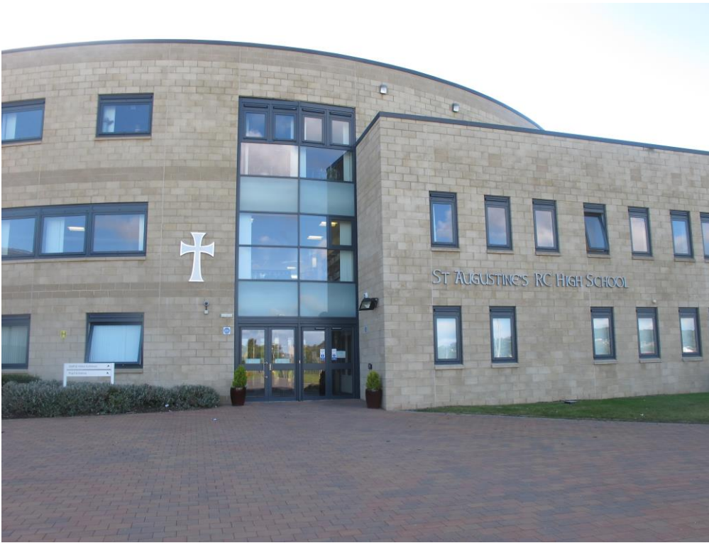
The front entrance
