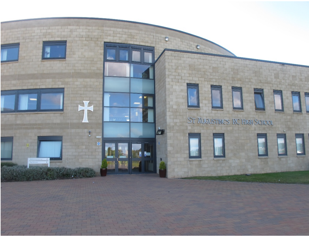
The front entrance
